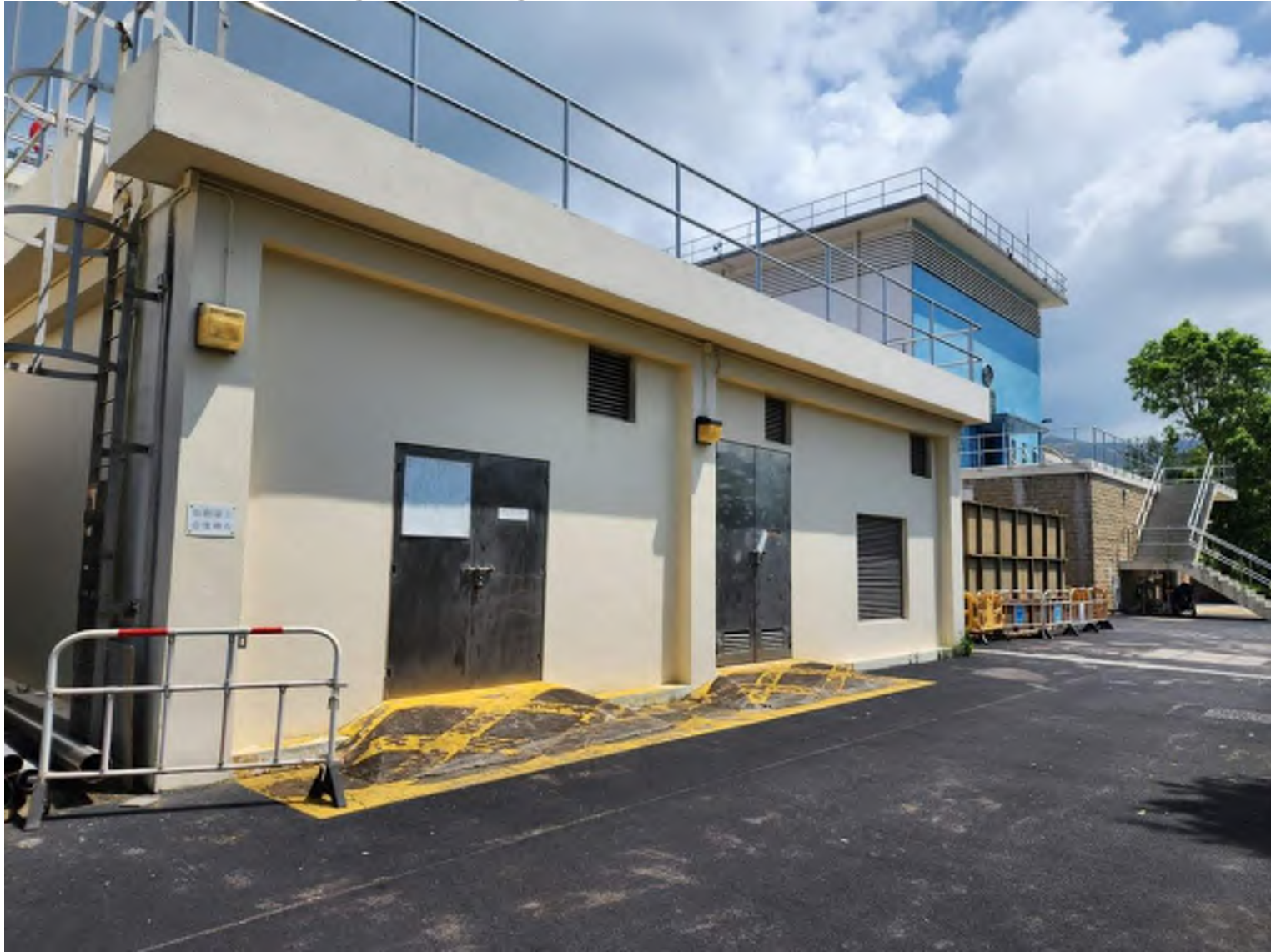
FIGURE 7 Site Photo 2 - Existing Pumping House
