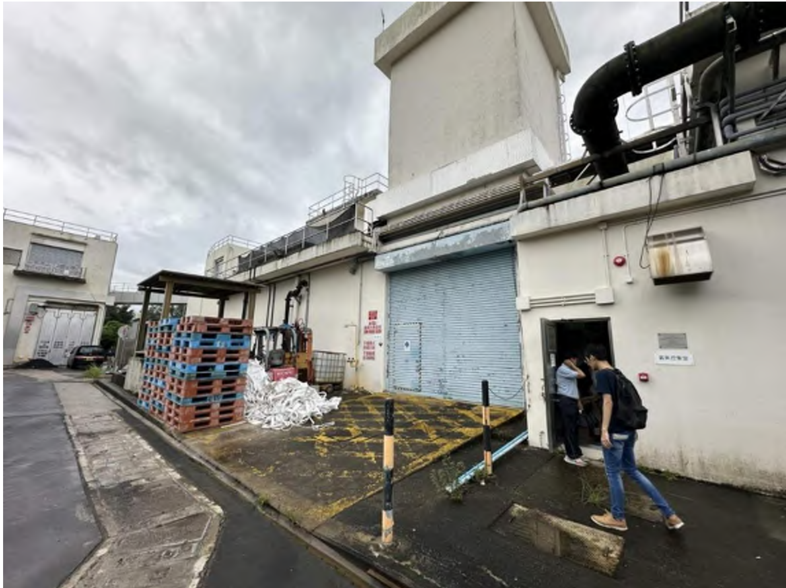
Site Photo 7 - Existing Chlorination House (Not in Used)
