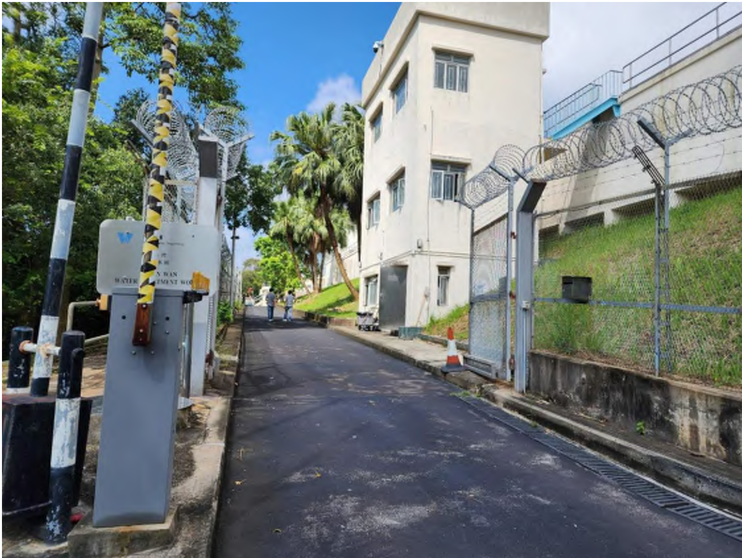
Site Photo 1 - Existing Main Gate to TWWTW
