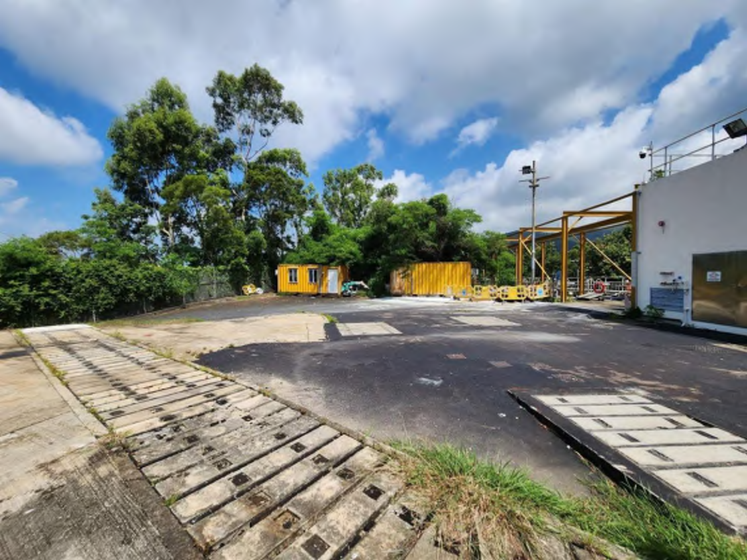
Site Photo 12 - Existing Access Road and Washwater Recovery Tanks
