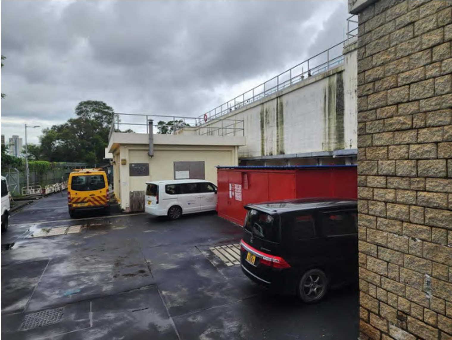
Site Photo 3 - Existing Dangerous Good Containers and Pumping House
