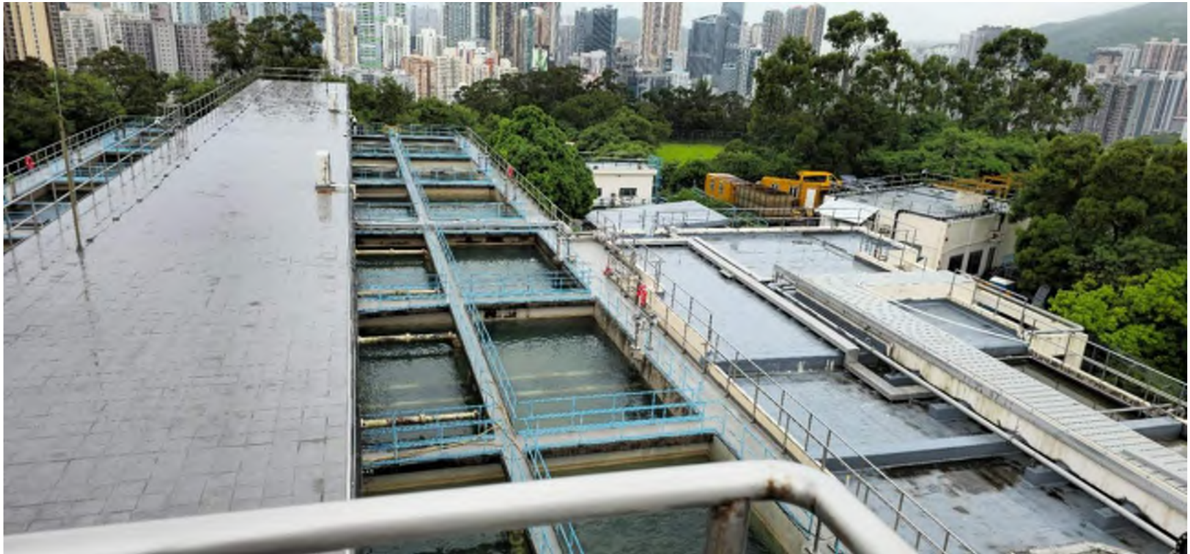
FIGURE 19 Site Photo 14 - Existing West Wing
