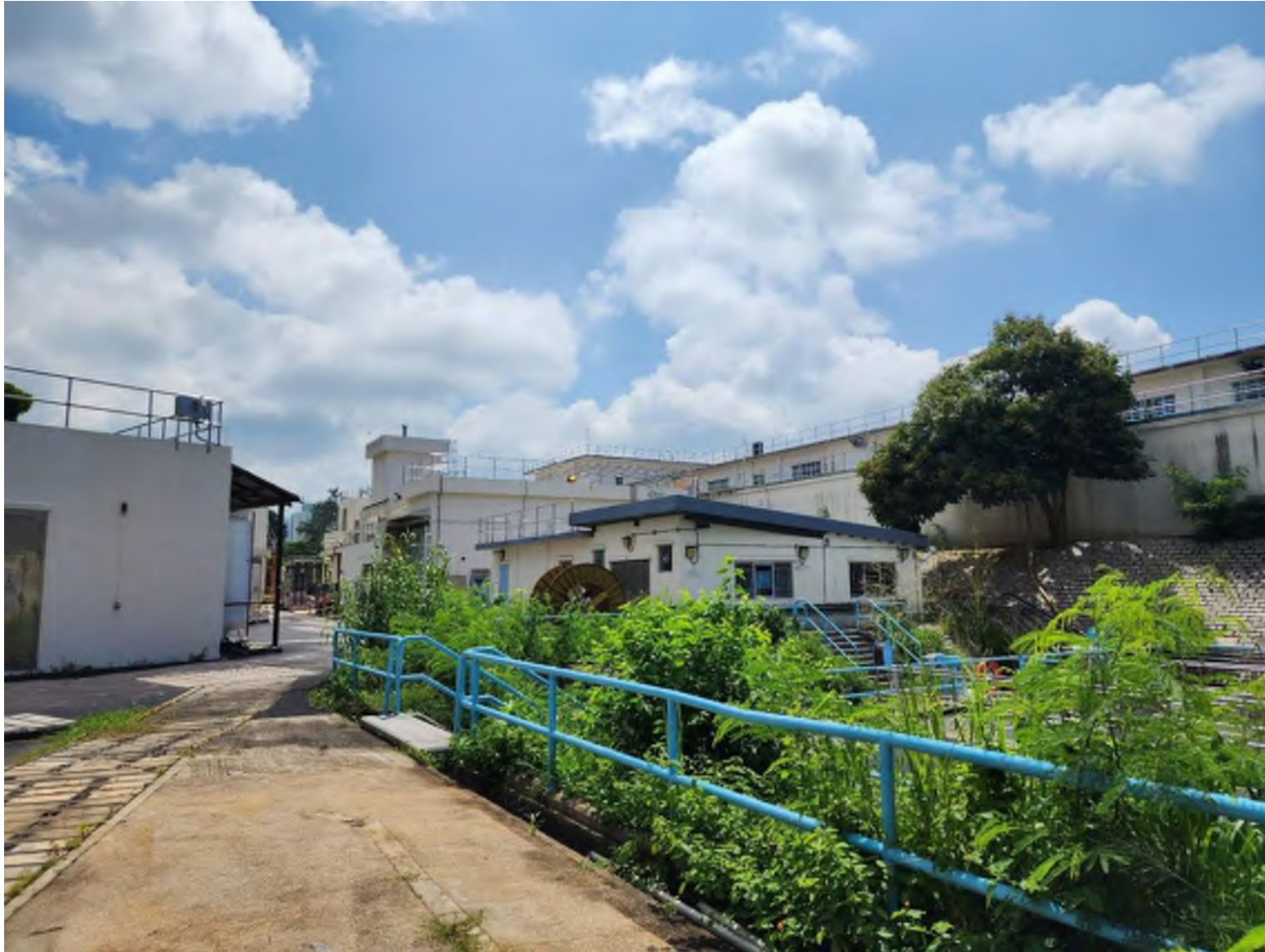
Site Photo 11 - Existing West Wing and Sludge Holding Tanks
